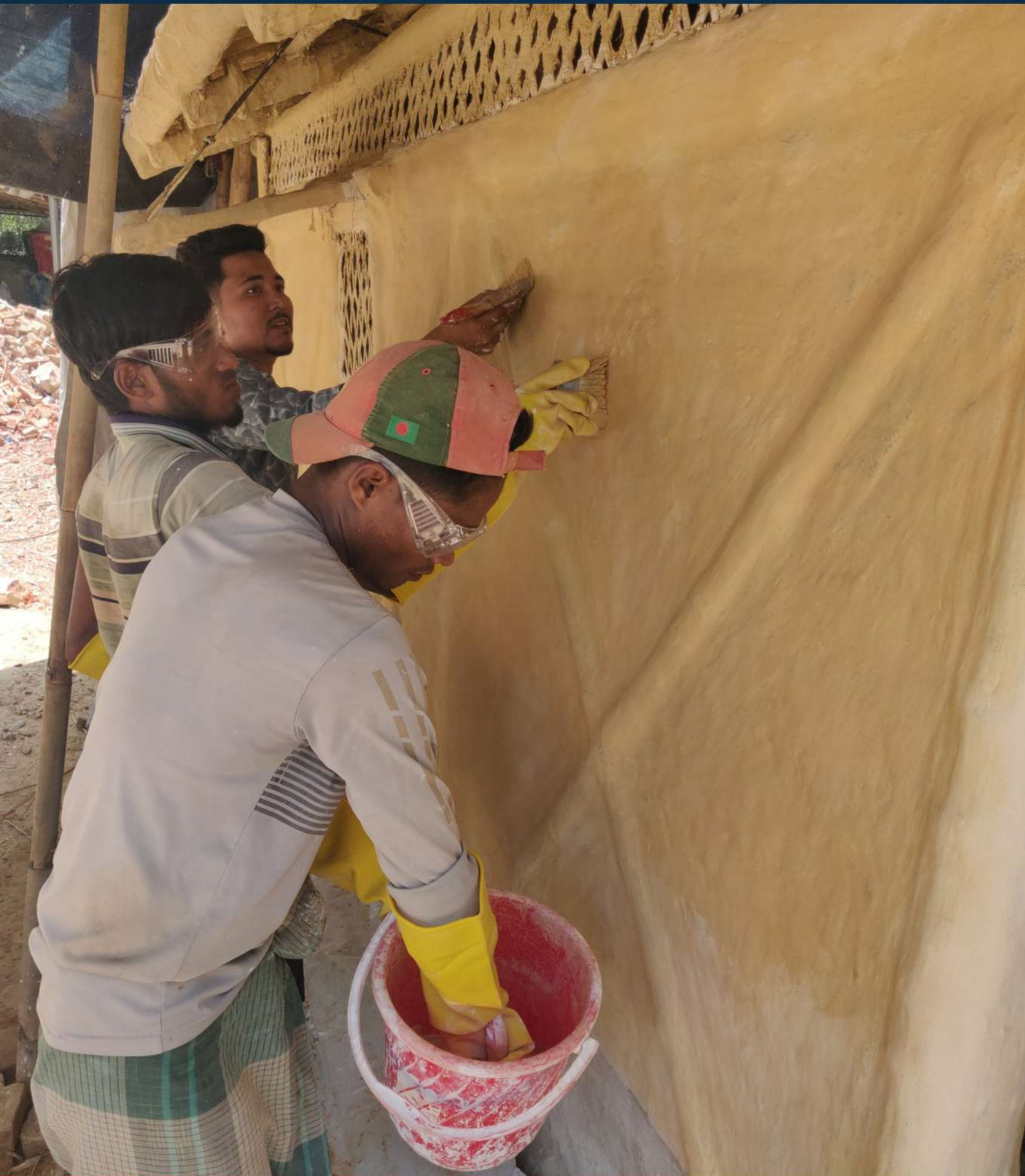
Lime Stabilised Soil Plastering of a shelter in Cox's Bazar
