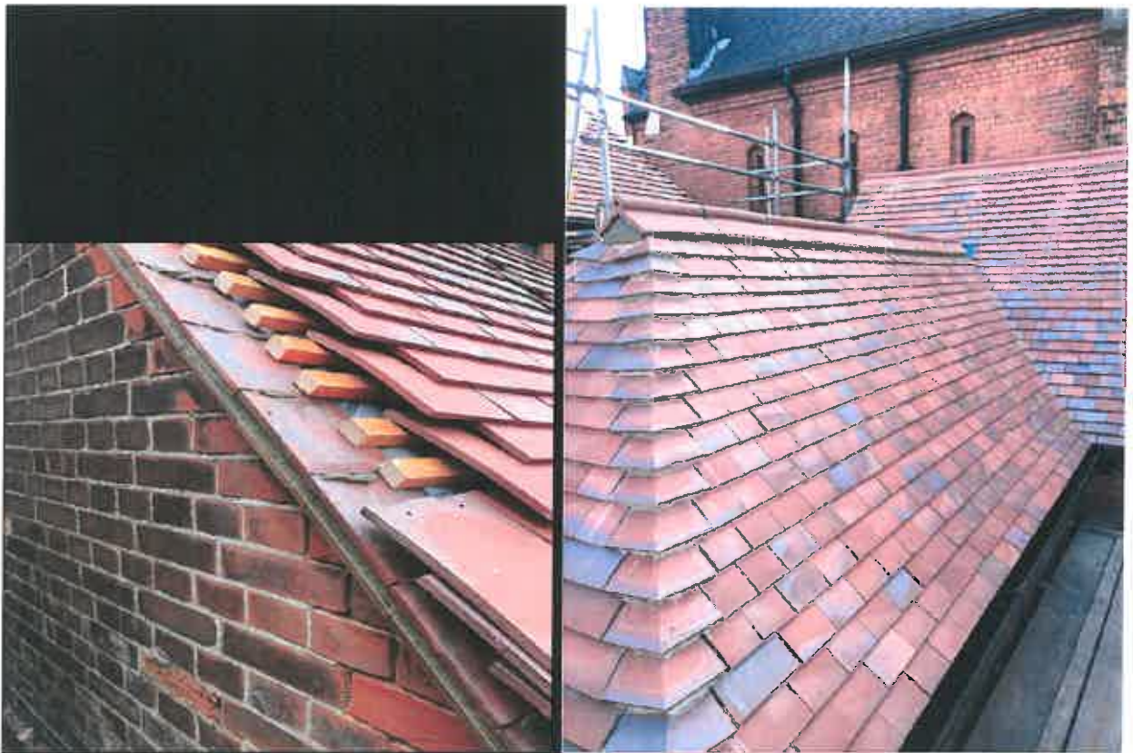
New Roof structure and roof coverings
