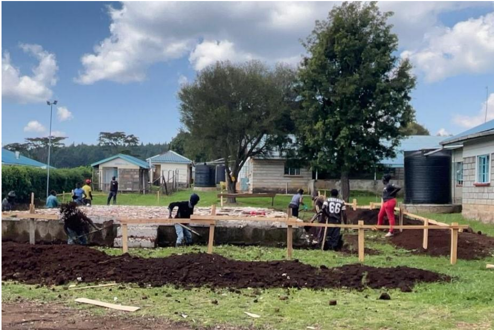
Starting construction of the new Trauma Unit at Londiani Hospital
