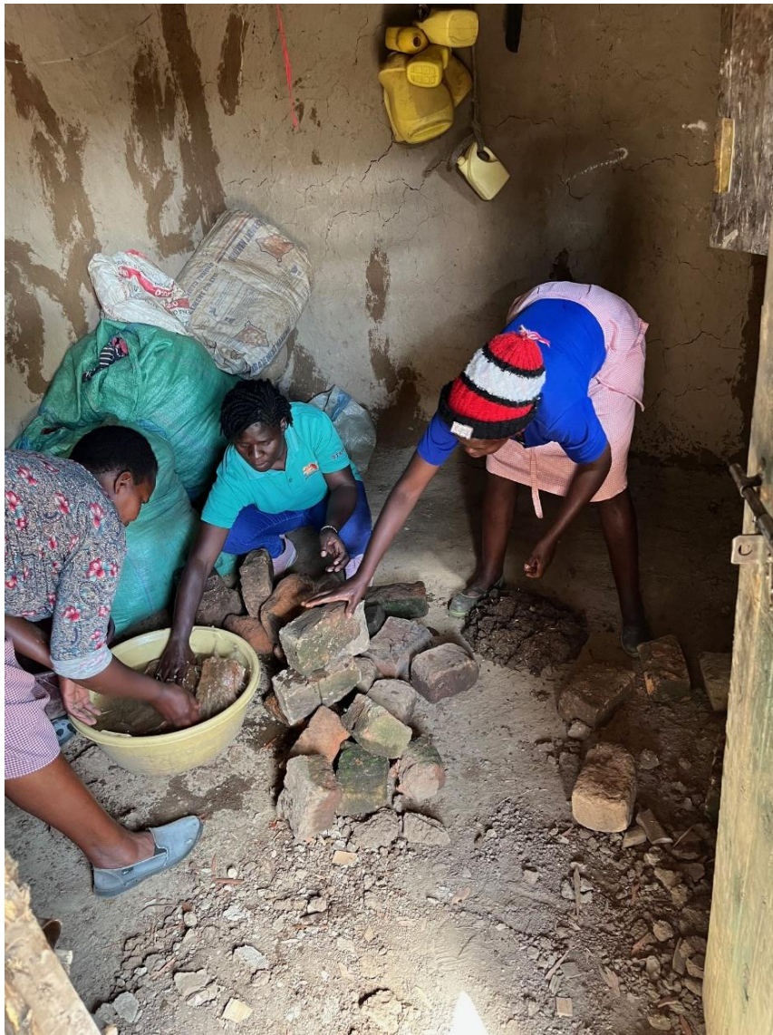
Constructing a smokeless stove – the “one hour miracle”
