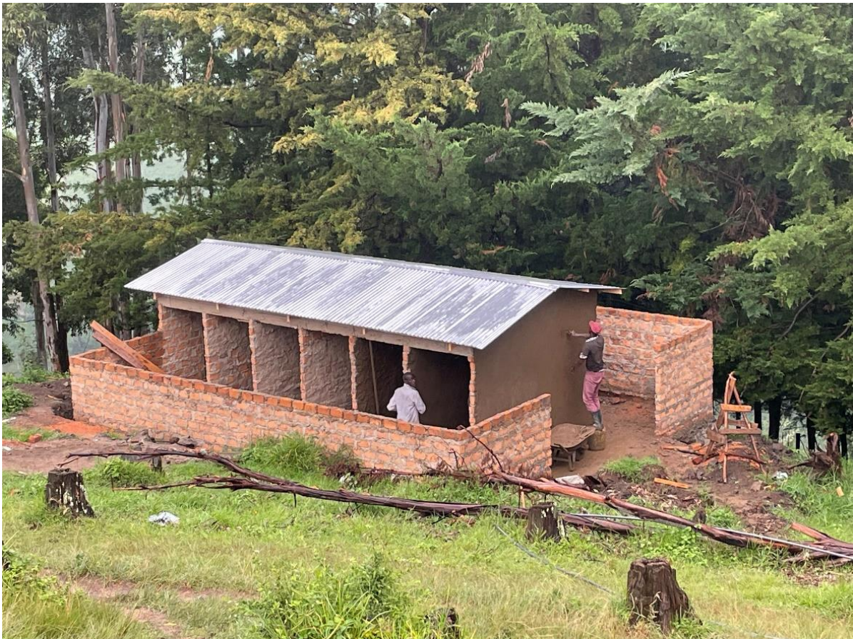
Latrine blocks under construction at Magire primary School
