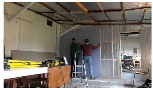
Hall refurbishment in progress
