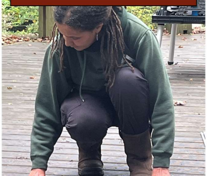
October 2024 Making safe the Raven's Nest with Groundwork London
