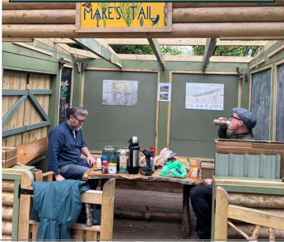
April 2024 Replacing the leaking roof on the Mare's Tail Cabin
