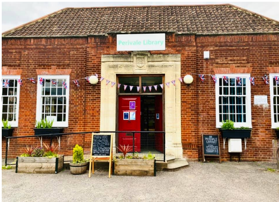
ABOVE – PERIVALE LIBRARY FROM THE OUTSIDE
