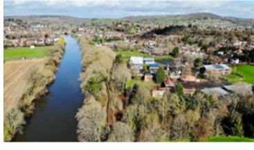
An image taken from a drone, during the survey, showing the school, town and the river Severn
