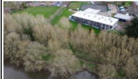
An image taken from our drone showing the school and the river Severn
