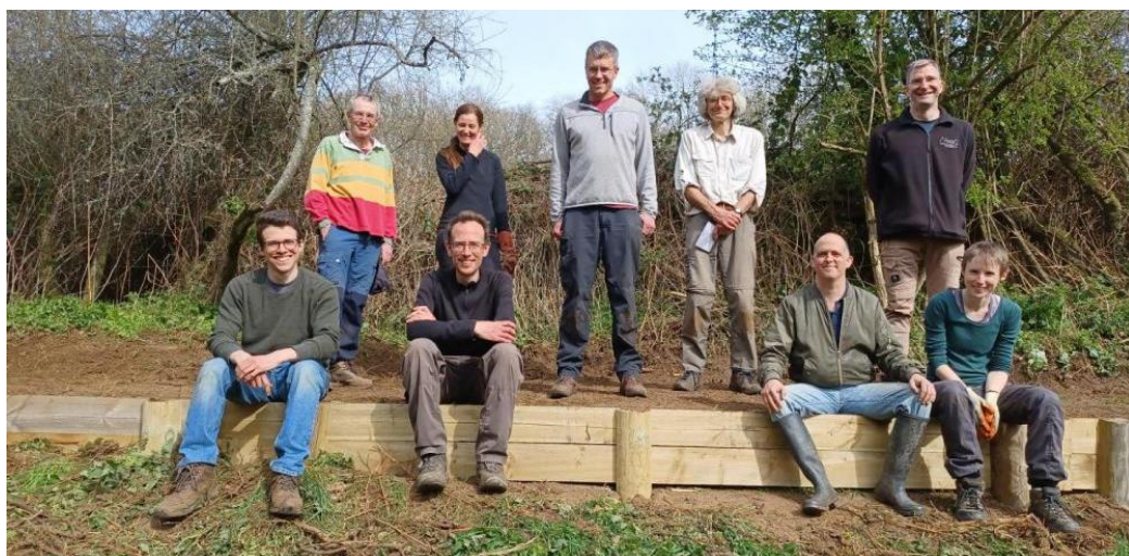
Revetment construction at Matthew Arnold Field, April 2022
