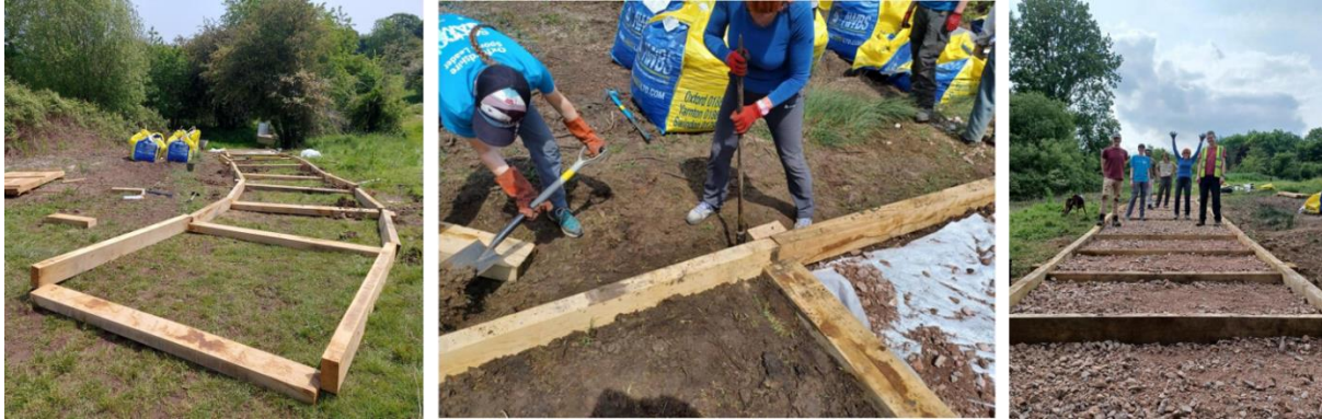
Sleeper step construction at Raleigh Park, Oxford on the 28 th May and 4 th June 2023. Steps were constructed to improve site access and prevent a muddy quagmire in winter in an area fed by natural springs.
