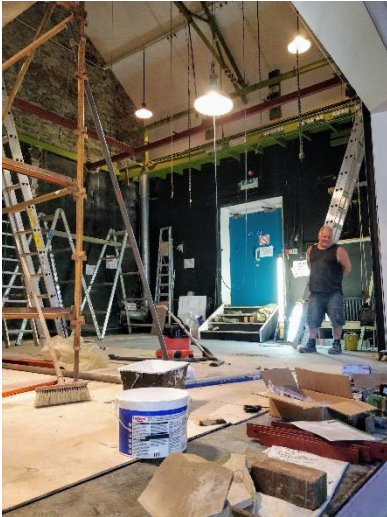
Fig 2 shows the work well underway to improve the safety and functionality of the stage in the Main Hall. A structural engineer's report had advised that the old gantry and plaster work to the rear wall was unsafe, hence the need for its removal. The hoists and winches were made redundant by the new scheme which installed new track for curtains and backcloths and fixed the new (mainly LED) lighting in place. The rear wall of the stage was cleared of plasterwork and the original stonework sealed and left on display from around 3 metres up to the ceiling.
