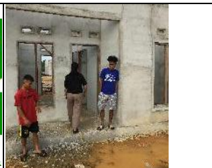
Inspecting the partially finished house
