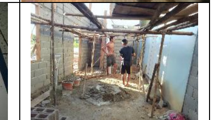
Work in progress on the extension
