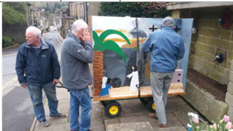
Members installing our Easter display in the Fox’s Head Well for The Pateley Bridge Town Council.
