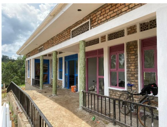
RSNF's newly constructed classrooms
