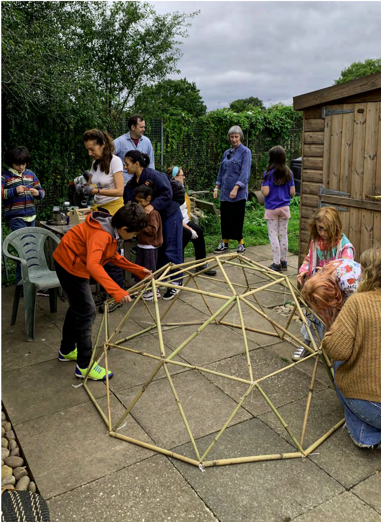
Geodesic Dome using two different lengths of bamboo, made up of six pentagons and ten triangles, ready for wire sound scores
