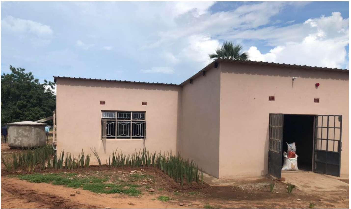
Photo: Kariba South Primary's solar-run Agricultural Hub Shop with rainwater harvesting demonstration system
