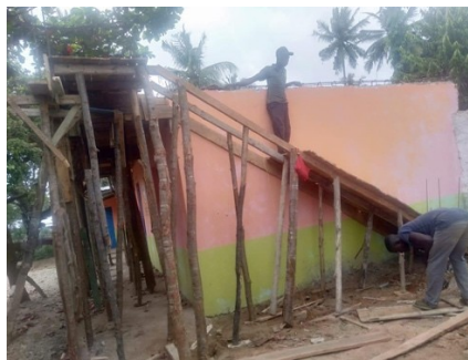
Photos of 1 st part of 1 st floor classroom extension completed September 2020.
