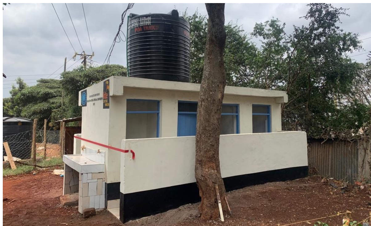
The completed toilet block.
