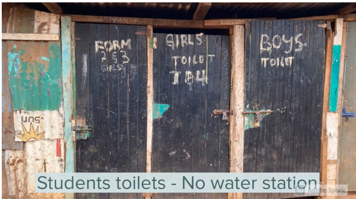
Student toilets at Silver Springs High School before renovation work began.
