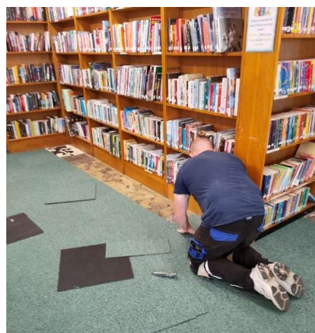
Laying the new carpet
