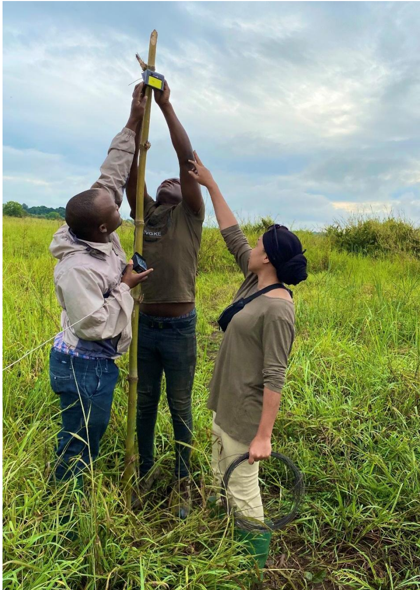
Setting up of the solar-powered strobe lights fence
