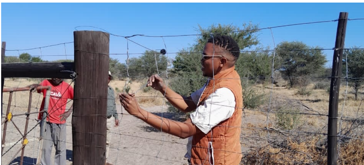
Photo 9: Efa Community Outreach and Education Coordinator, Mr Walona Sehularo, demonstrates connecting offset brackets to an electric fence.
