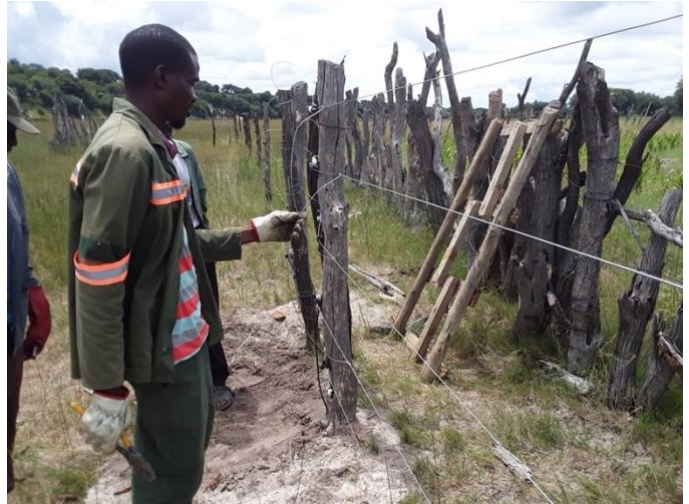
Photo 3: Efa Community Officer for Moreomaoto, Tathego Bolekanye, Installing an electric fence around a cluster farm.
