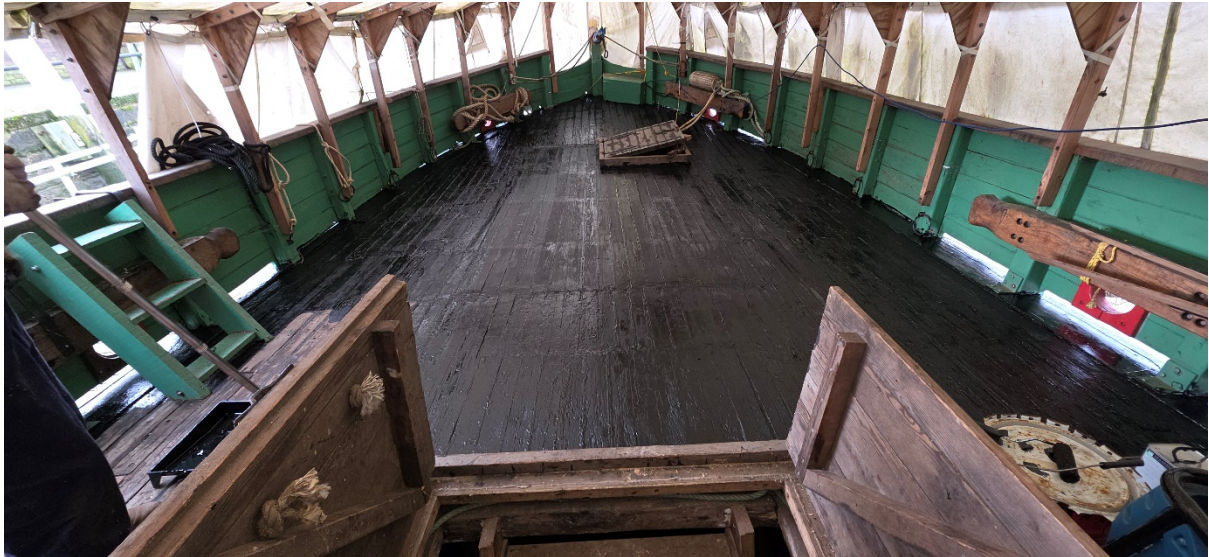
Deck repairs have been ongoing throughout the year
