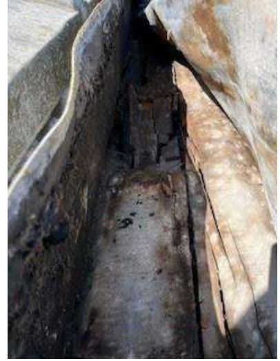
Looking west at rotten timbers.
