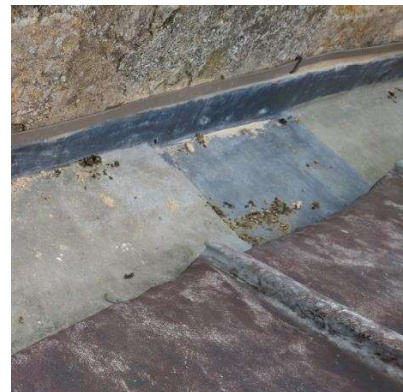
Repaired lead outlet and north Nave gutter and flashing.
