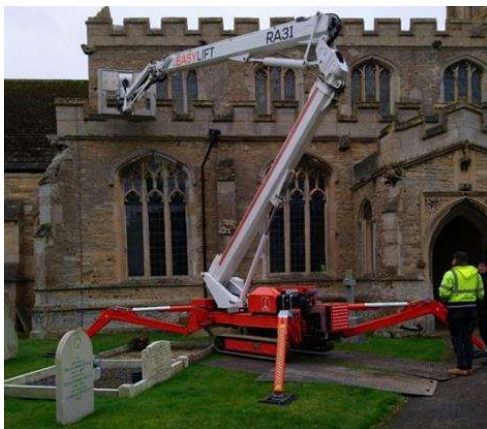
Installing the lightning protection upgrade.
