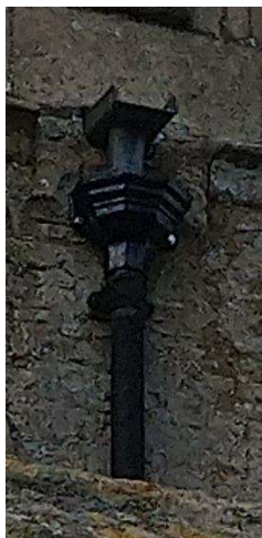
Repaired lead outlet and north Nave gutter and flashing.
