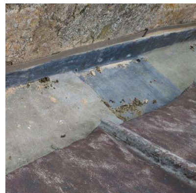
Repaired lead outlet and north Nave gutter and flashing.
