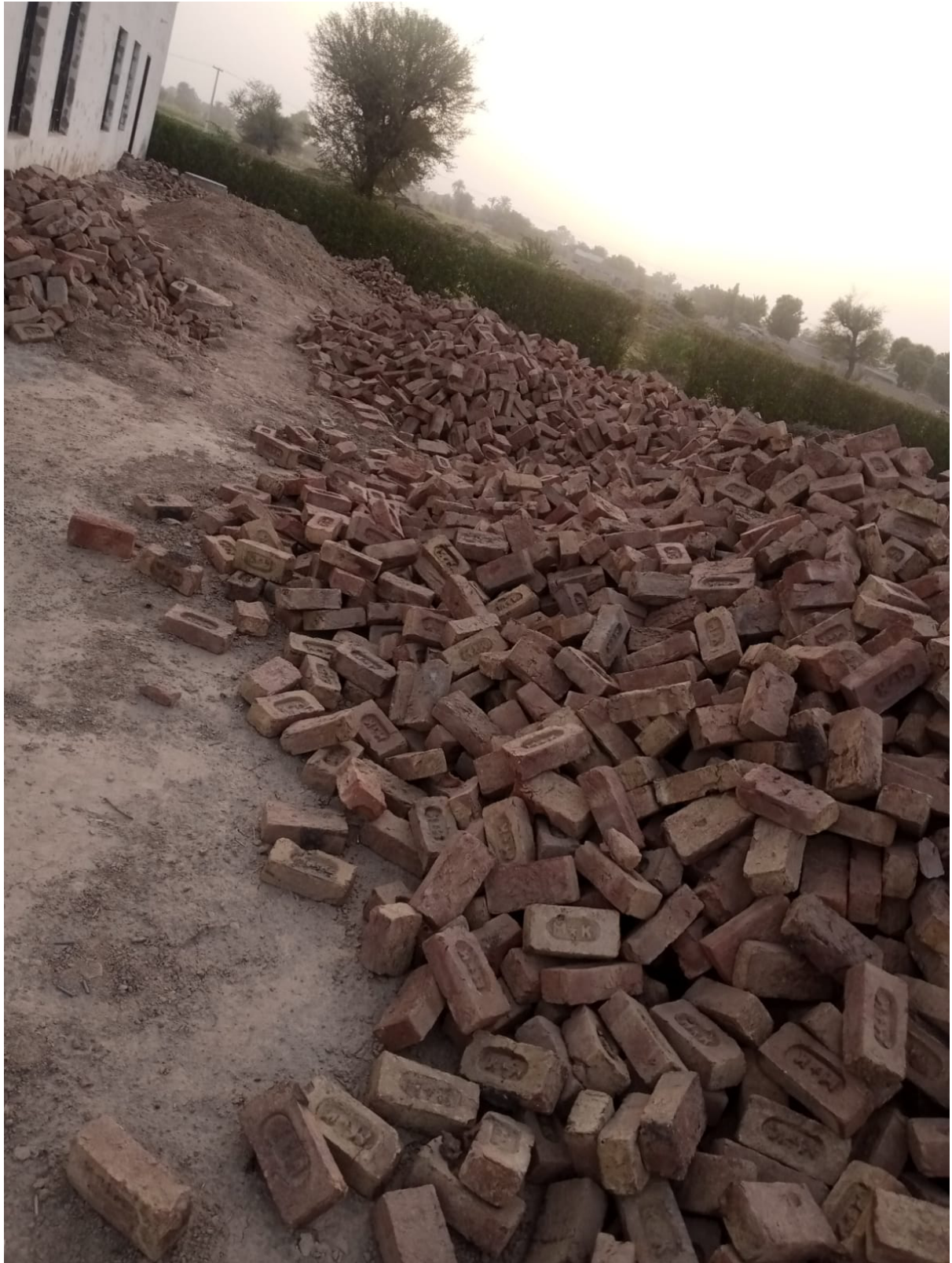
Figure 3/ Additional four rooms being constructed at 1st floor
