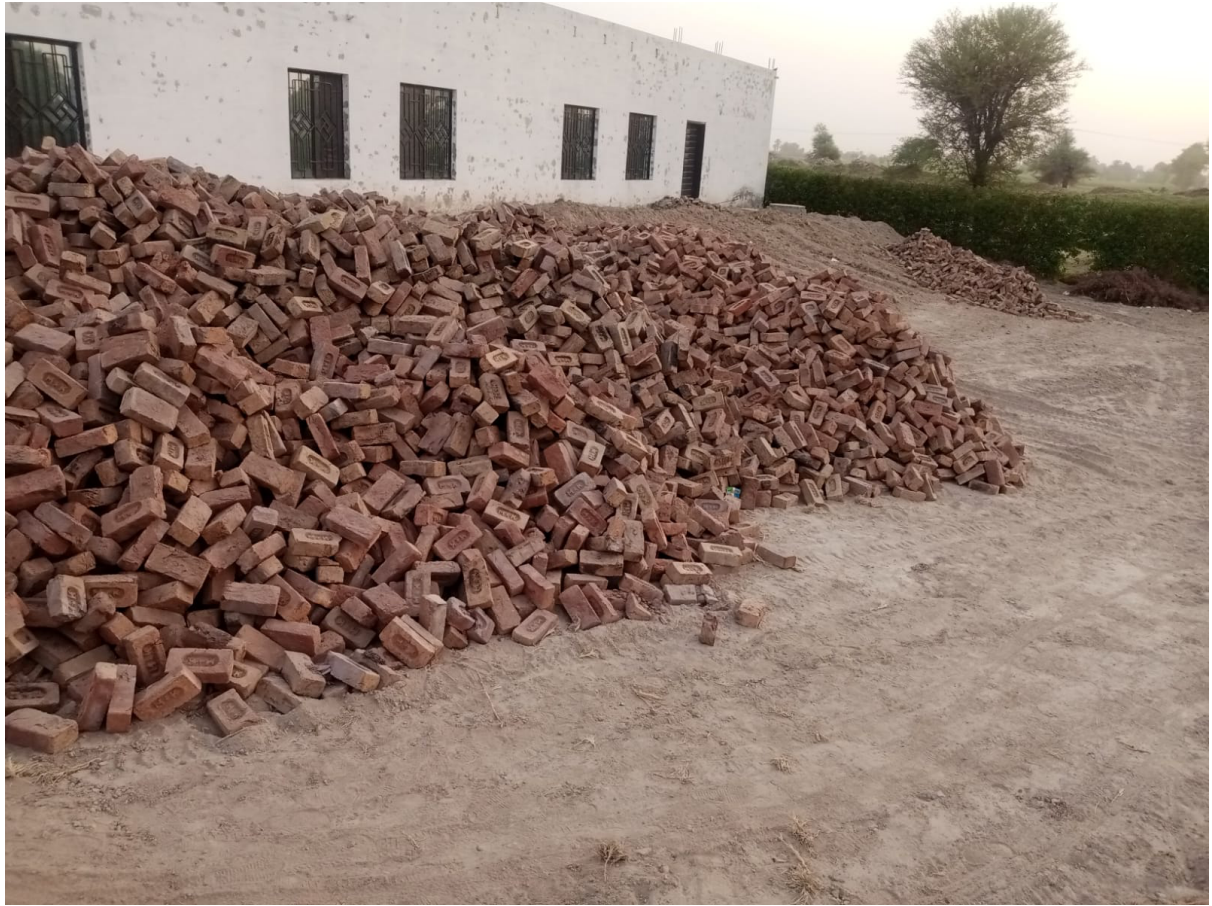
Figure 4/ Four rooms at 1st floor under construction
