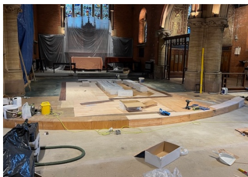
RE-ORDERING WORKS UNDERWAY
