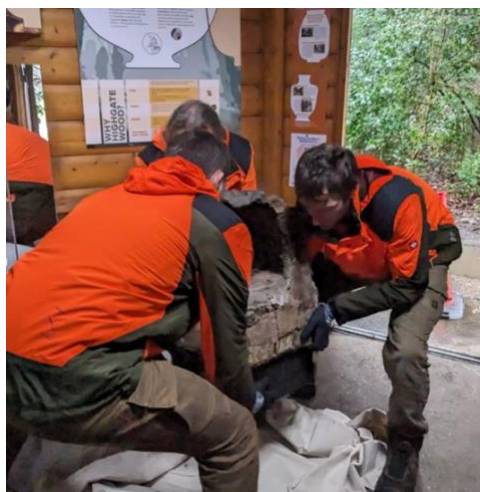
The Natural Building Centre team removing a kiln piece from the Highgate Wood information Centre
