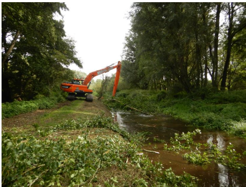
Big machinery placing tree ledges for flow deflection at the Alder Carr reach at West Stow, October 2022
