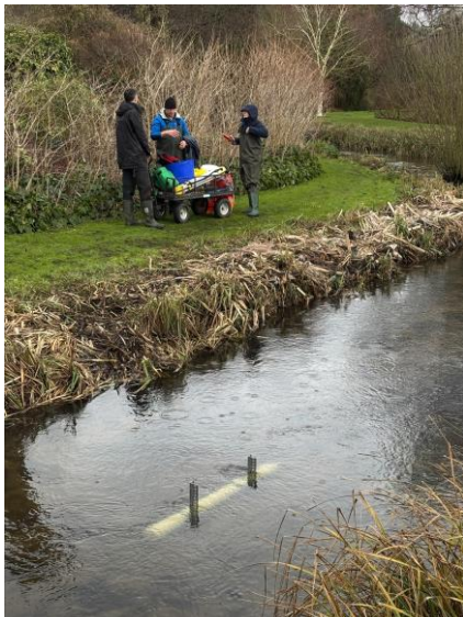
Installing a sediment collecting tube
