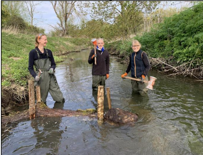
Another flow deflector installed
