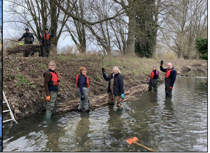
Making progress with the brush bundles
