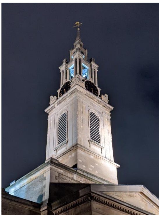
New floodlighting of St James tower
