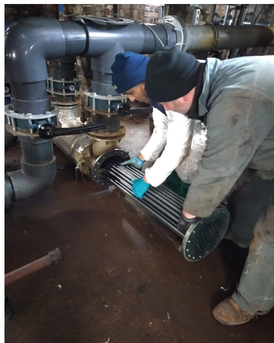
Calorifier Removal, Plant Room, January 2023
