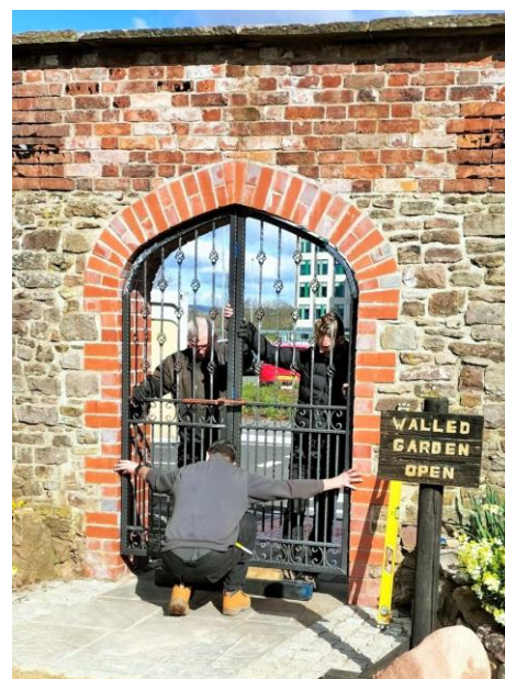
'Offering up' the new north gates
