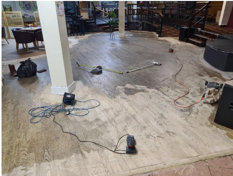
Picture 7 – Sanding off in progress
