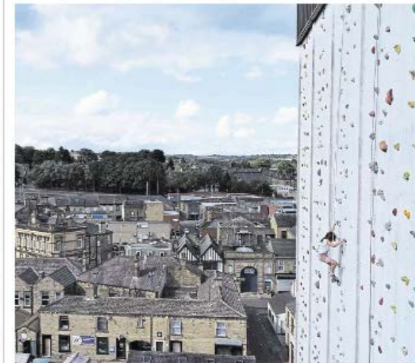
A climber tackles ROKTACE, the UK's highest outdoor man-made climbing wall, located at ROKT in Brighouse. It has not operated since before the Covid-19 pandemic and profits from all climbs yesterday went to the ROKT Foundation climbing charity www.roktfoundation.co.uk .
