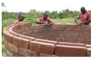
ISSB Rainwater Tank construction. Credit: www.hytuganda.com
