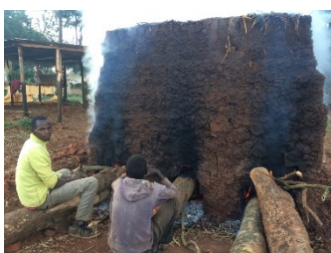
Traditional brick firing using tree trunks Credit:KEEP
