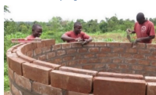
ISSB Rainwater Tank construction Credit: www.hytuganda.com
