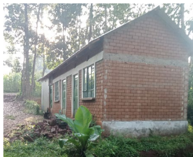
Completed Guest Houses
