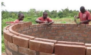
ISSB Rainwater Tank construction Credit: www.hytuganda.com
