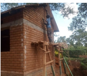
Finishing the gables
