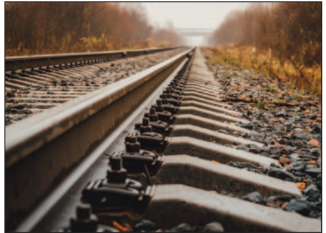
Supporting the reinstatement of the Okehampton to Exeter passenger rail service
