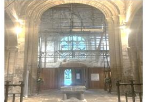
Internal Church Repairs
