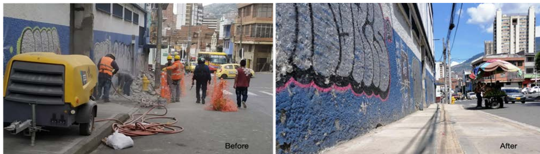
Works in Medellin, Colombia – widening the sidewalk
