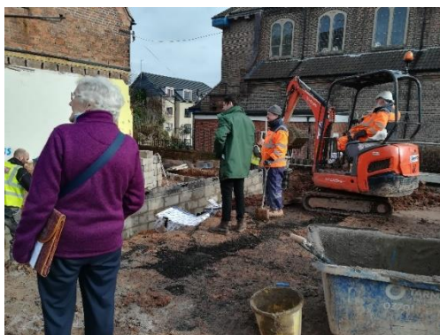
Sister Margaret monitors building work progress at Carlton property
