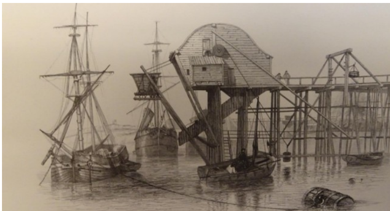
and showing how the wagons delivered coal through special machinery to waiting colliers for transport to London..
