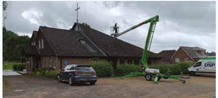
Fixing the leaking roof at Bearsted
