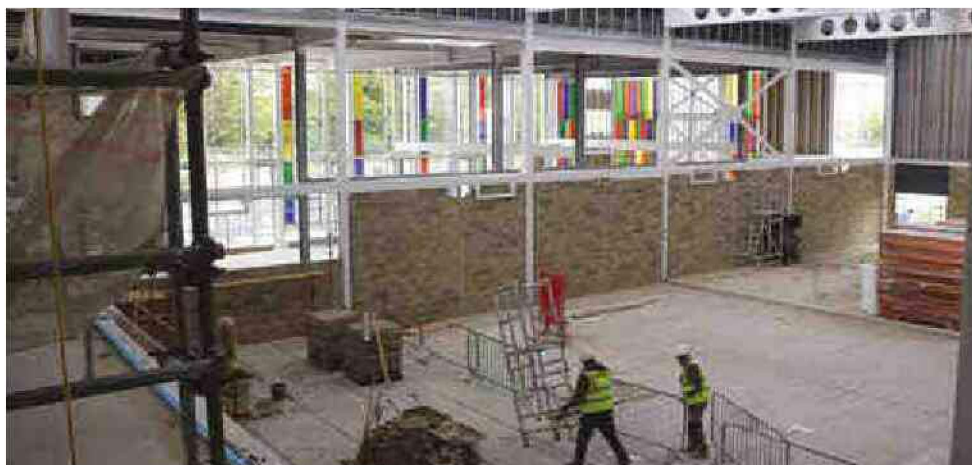
Building of the new St John Fisher School in Chatham
