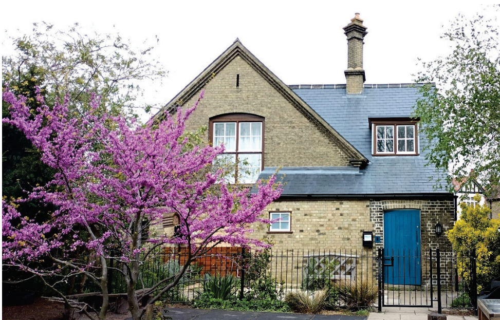
The refurbished Old School building where the Parish Office is now located
