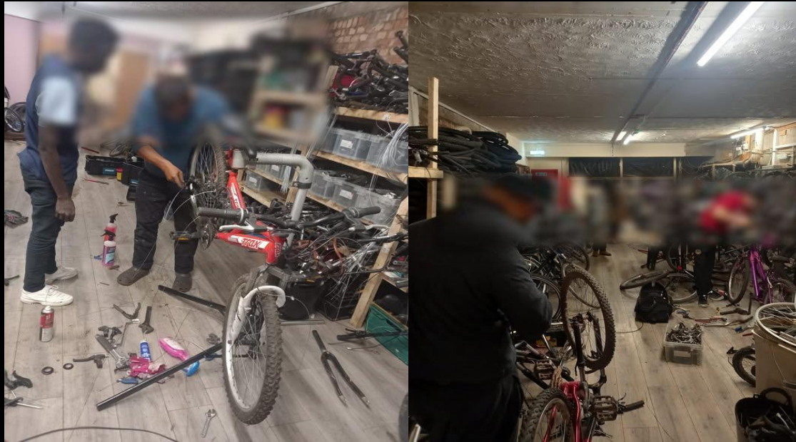
In process of creating new bike shop with RAS volunteers learning new skills and building their community. It now has a toilet, washbasin and small kitchen.
