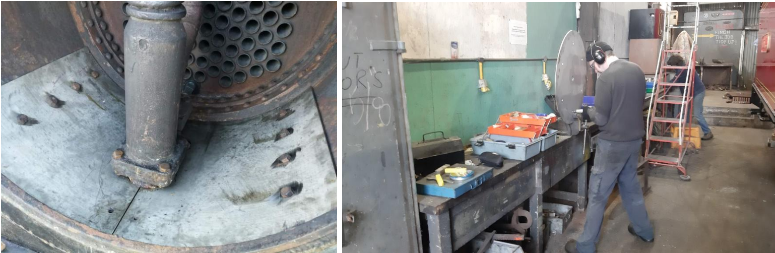
Gelert's new smokebox floor (left) and baffle plate (right) being made and fitted by our trustees and volunteers. (photos: Myles Jones)
