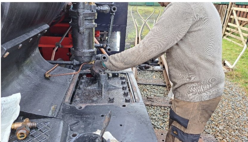
Photo – Gelert's left hand cylinder cover being removed for inspection
