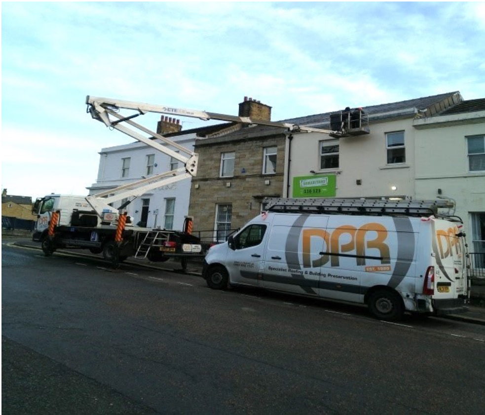
ROOF MAINTAINANCE AT THE BRANCH
