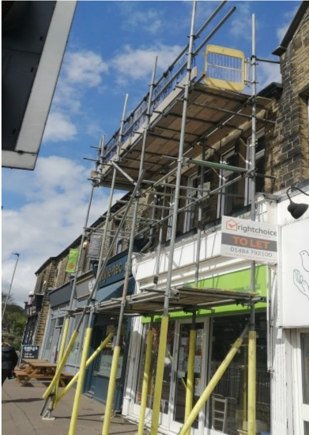
Repairs To The Shop Roof
