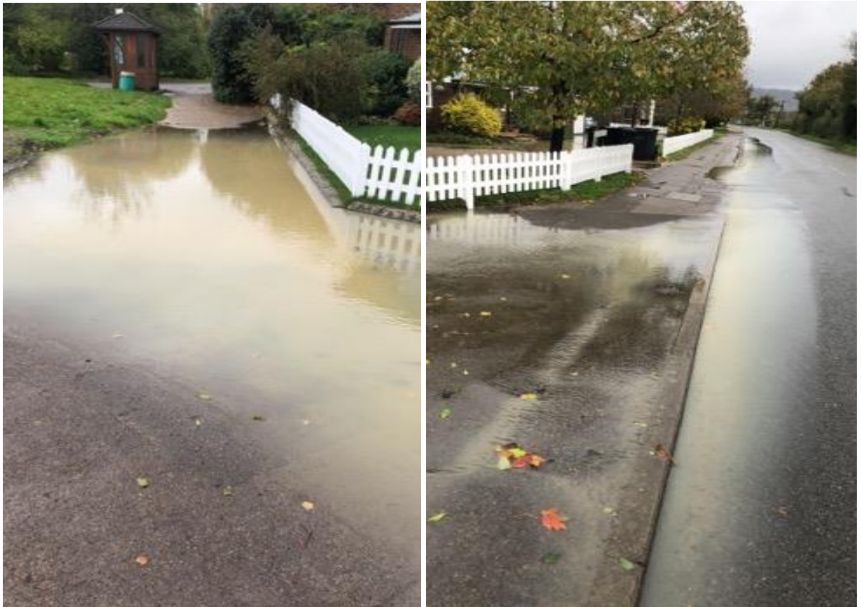
BERT has been reporting the blocked drains at Brockham Row for over five years and requesting action from Surrey County Council
