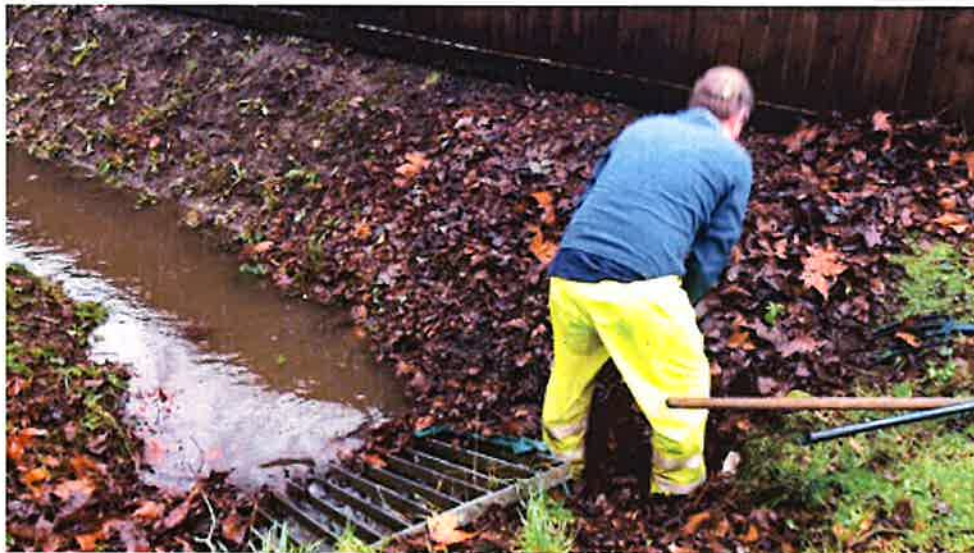
The grill in Wheelers Lane was heavily congested with litter at the seat of the blockage
