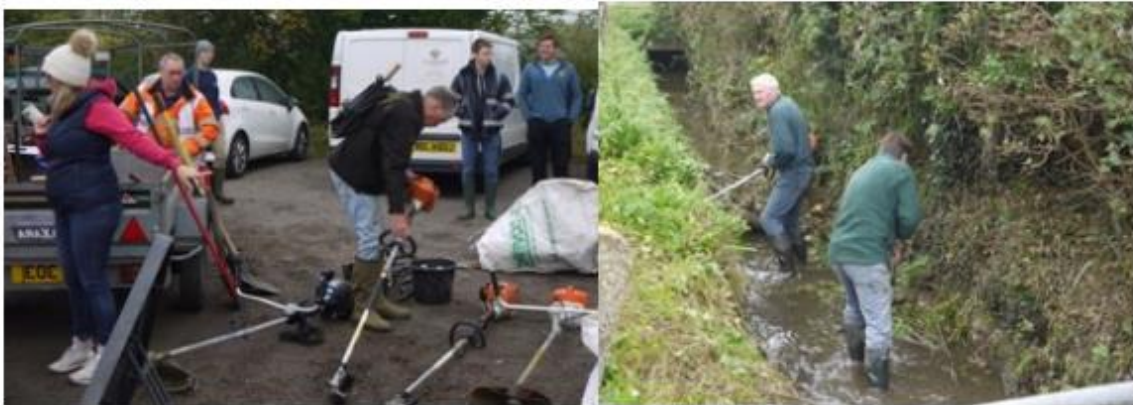
In February a team of volunteers utilising some significant plant loaned by a local farmer undertook a range of ditch clearing actions across the village watercourses
