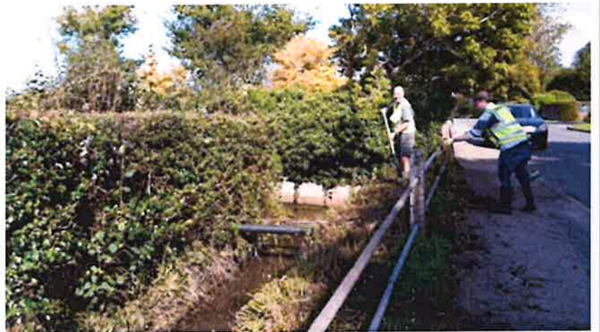
Main drainage ditch by pavilion
