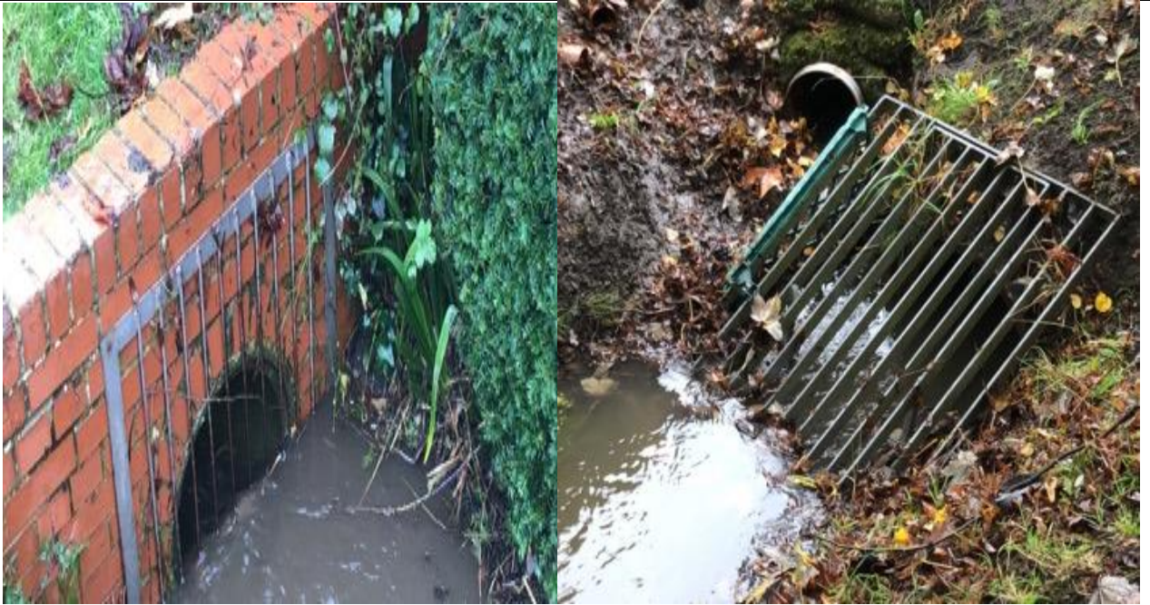
BERT volunteers cleared the grills and culverts at Wheelers Lane.
