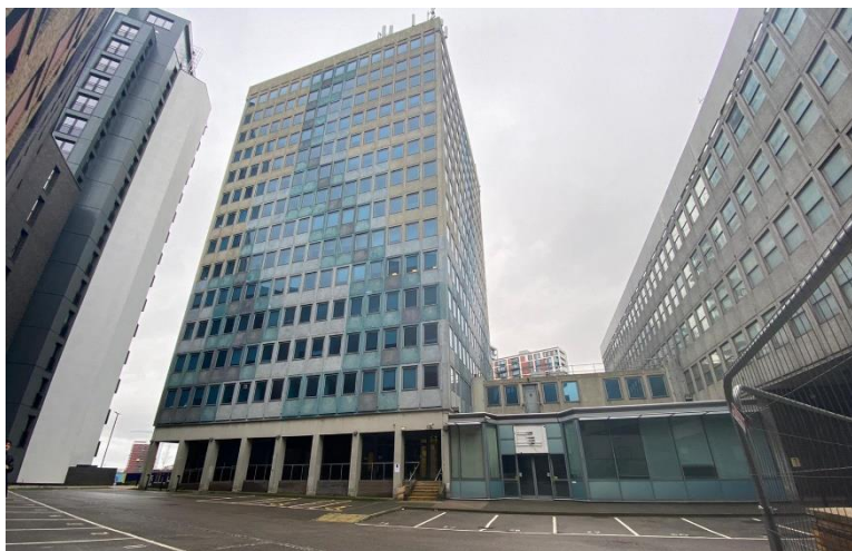
SET Woolwich, west tower, January 2021
