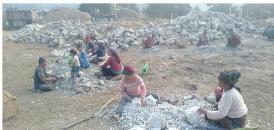
Local People Creating Aggregate from Stone
