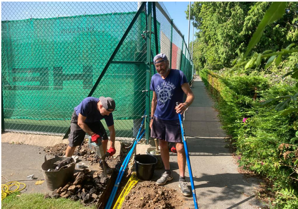
Paul Thomas and John Callaway digging a trench for the court 4 LED lights wiring
